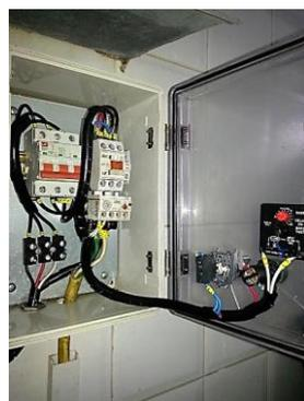
**Figure 21. Level Control dash mounting**
