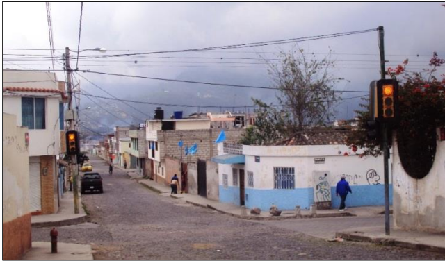
Figure 17. Junctions system installed on the public highway
