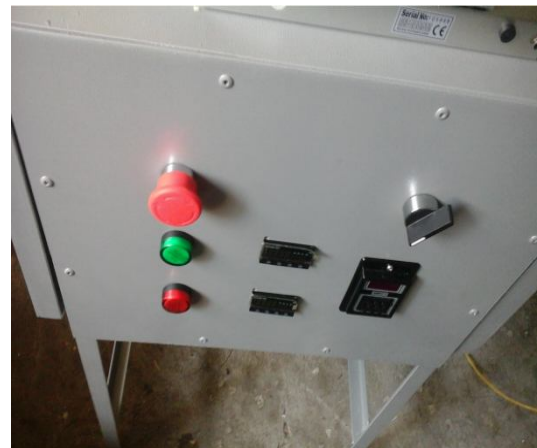
FIGURA 9. Panel de control
