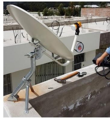
Fig 10. Assembly and fixing the antenna
