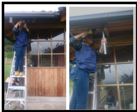
Figure 6. Implementation support Antenna Litebeam M5-23, Protective Forest.
