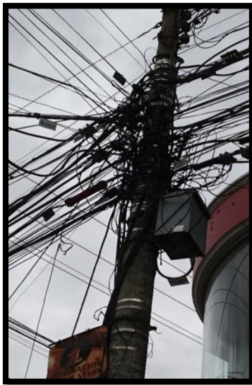
Figure 4 Saturation Cables in Avenue Alfredo Pérez Guerrero post and Simón Bolívar
