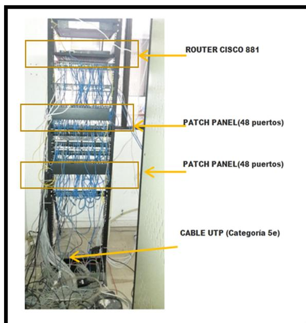
**Figure 5.** Rack located in the equipment room front view
