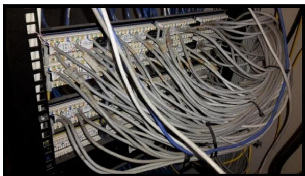
**Figure 4.** Patch panel 48 ports located in the telecommunications room
