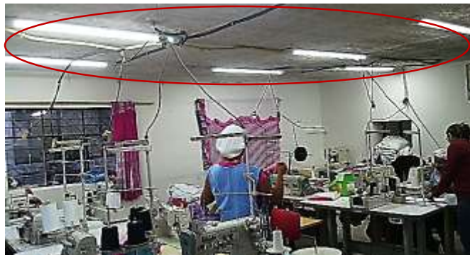
Photo 2: IMPROVEMENT OF LIGHTS
