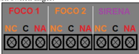
Figure 15. Connecting electrical devices in the cabinet
