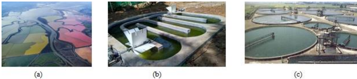
Figura 2. 2. Biorreactores abiertos [10], (a) Open ponds, (b) Raceway ponds, (c) Tanques circulares
