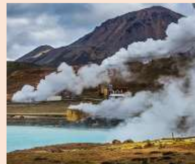
C Geothermal energy
