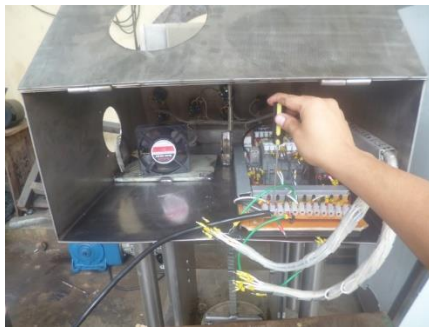
Figure 19 Mounting the control board
