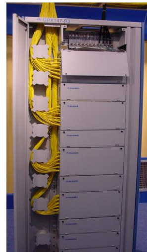
Gabinete ODF GPX147-R2 (800mm(W)×300mm(D)×2200mm (H))
