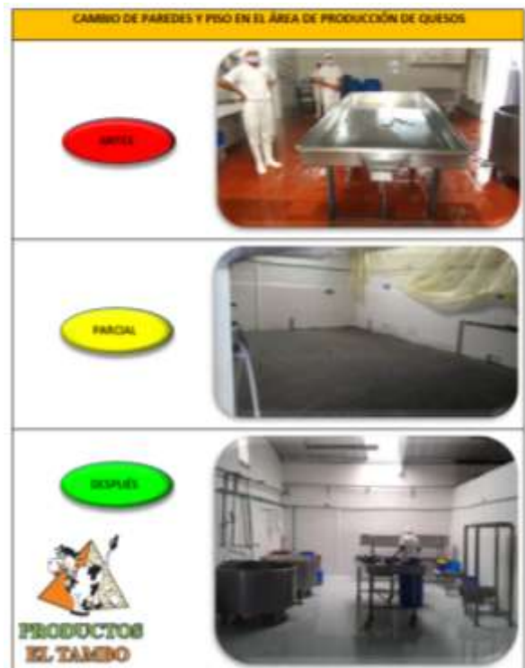
Figure. 3. Changing walls and floors in the area of production of cheeses
