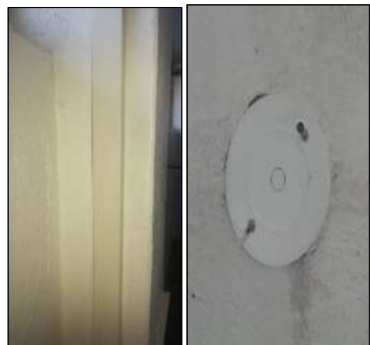
Figure 18. Electrical Installations after deployment Source: Company "Dairy Products Yaznan". Developed by: Mariela Cepeda
