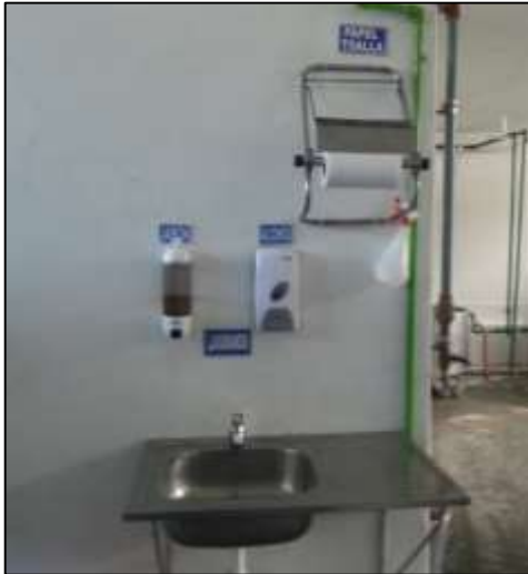
Figure. 4 - Deployment of washbasin within the area of production Source: Company "Dairy Products Yaznan". Developed by: Mariela Cepeda
