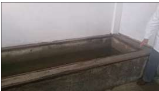
Figure 15. Water storage tank recycled Source: Company "Dairy Products Yaznan". Developed by: Mariela Cepeda
