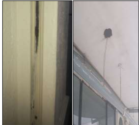
Figure 17. Electrical installations before deployment Source: Company "Dairy Products Yaznan". Developed by: Mariela Cepeda
