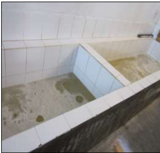
Figure. 23. Salero old fact of tile Source: Company "Dairy Products Yaznan". Developed by: Mariela Cepeda
