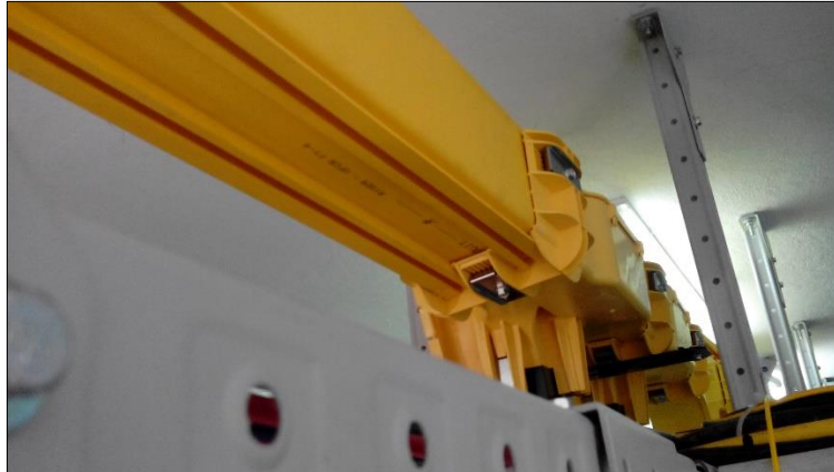
Figura 15. Fiber Runner existente
