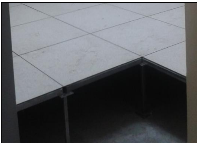
Figure 18. Technical floor installed Source: Project Design Data Center FICA
