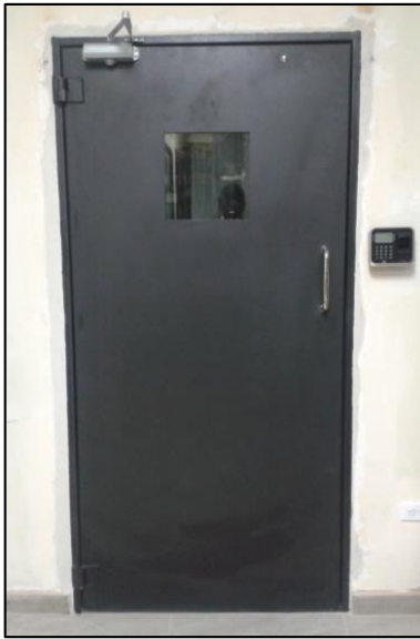
Figura 21. Security door Data Center Source: Project Design Data Center FICA
