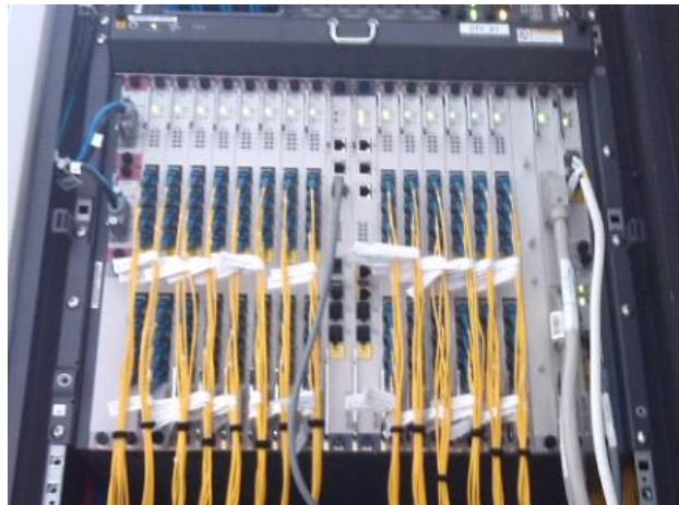
Figura 55. OLT Huawei MA5600T
