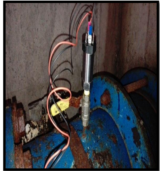
Figure 18. Connecting the pressure sensor to the main drinking water line
