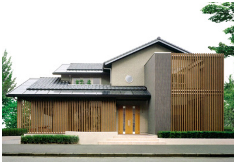
Figura 25.8: Building integrated PV. (Source: Sanyo Homes Corp.)
