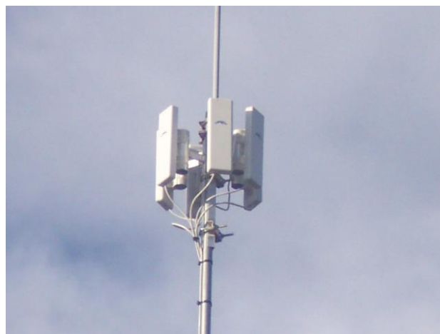
Figure15: sectorial Antennas
