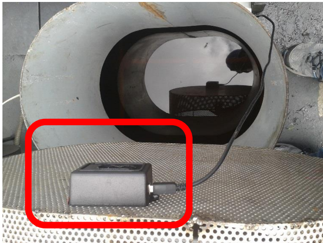
Fig. 28: Installation of water level survey
