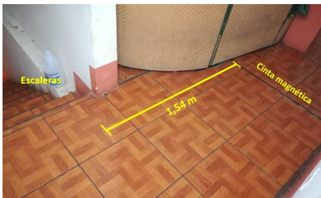
Fig. 54. Magnetic tape installed at 1.54m from the stairs Source: Prepared by the author
