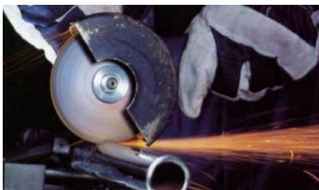
FIGURE 23: Manual cutting of steel Source: Authors
