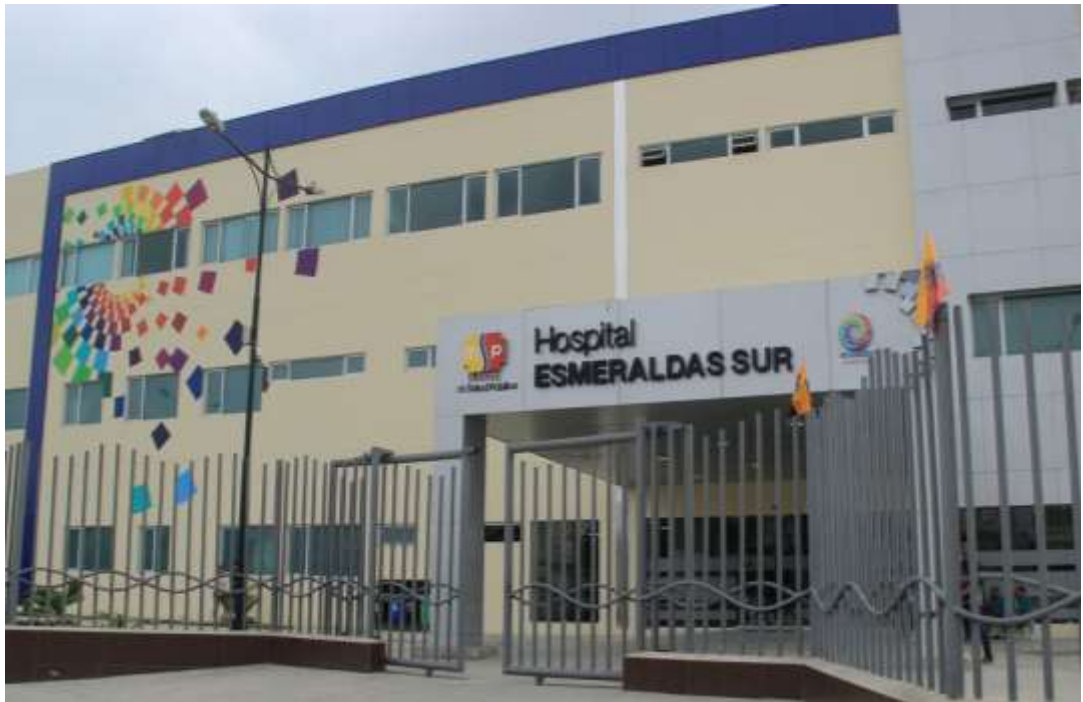
Figura 1. Hospital General Esmeraldas Sur
