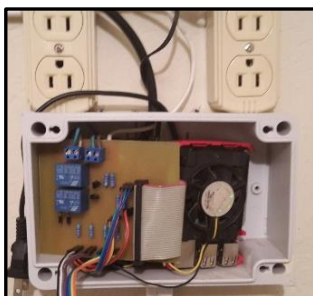
Figure 24. Installation of the plate Raspberry Pi 3 with its fan. Source: Authorship
