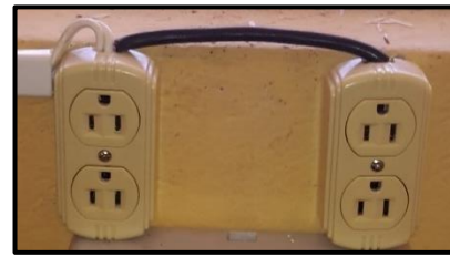
Figure 15. Installing the power supply for electronic devices. Source: Authorship
