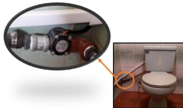
Figure 19. Installing the water flow sensor. Source: Authorship
