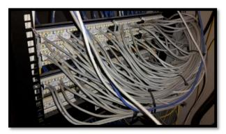
Figure 4. Patch panel 48 ports located in the telecommunications room
